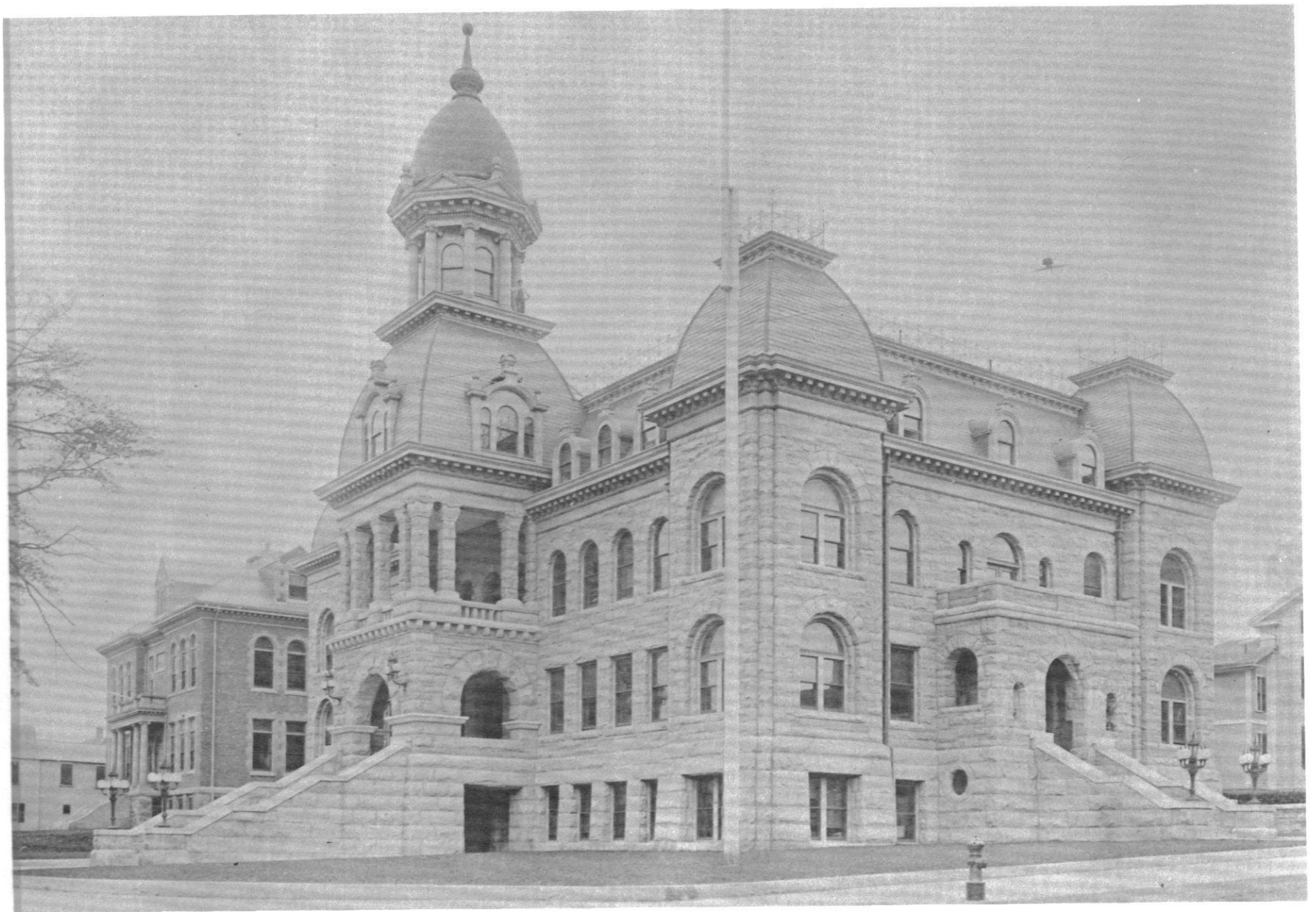
Figure 36: Newport City Hall, 1898-1900, altered 1927; photograph, c. 1900; 41 Broadway.
