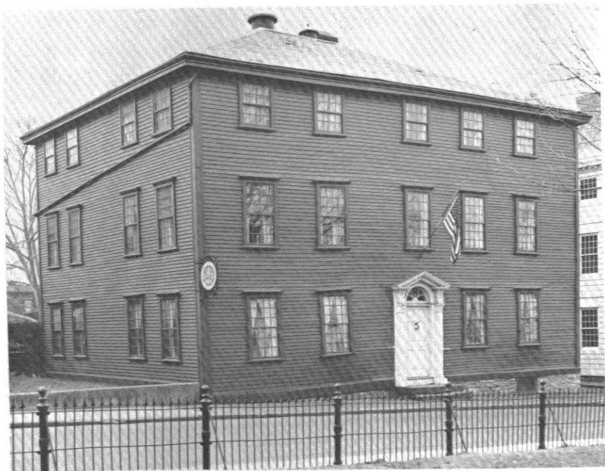
Figure 18: Joseph Rogers House (Headquarters for The Preservation Society of Newport County), c. 1790; 37 Touro Street.
