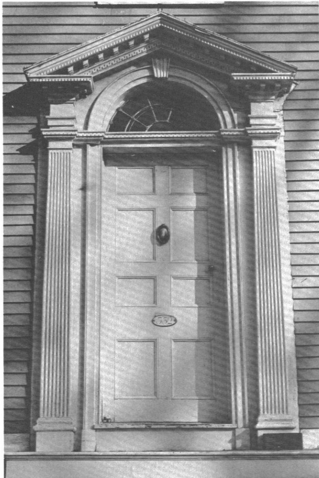
Fig. 15: Samuel Durfee House (1803), 352 Spring Street; front entrance.
