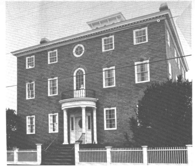
Fig. 17: Samuel Whitehome House (1811), 414-418 Thames Street, after renovation.
