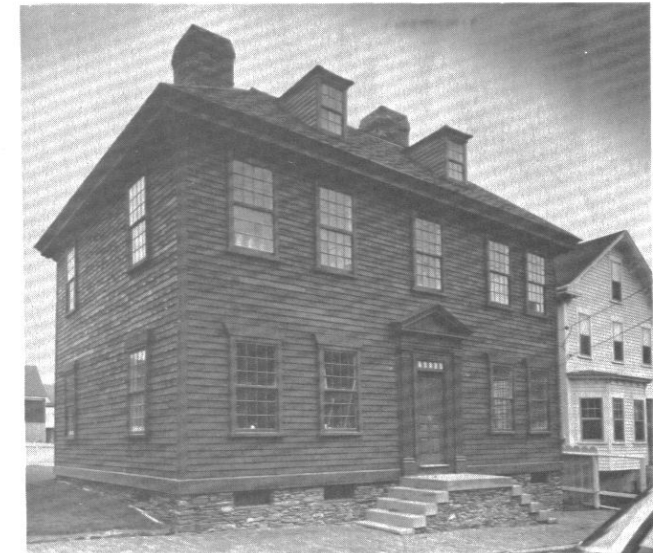
Fig. 12: Edward Cole House (c. 1760), 29 Howard Street.
