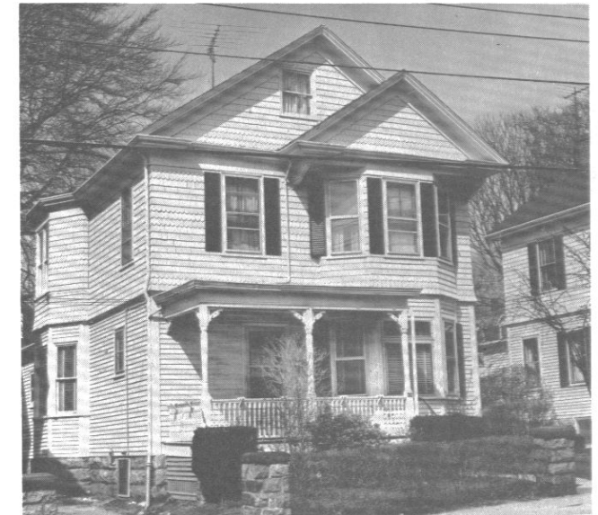
Fig. 47: Sullivan House (c. 1898), 30 Narragansett Avenue.
