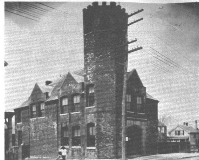
Fig. 34: Former Fire Station #6 (1891), 595 Thames Street; tower now removed.
