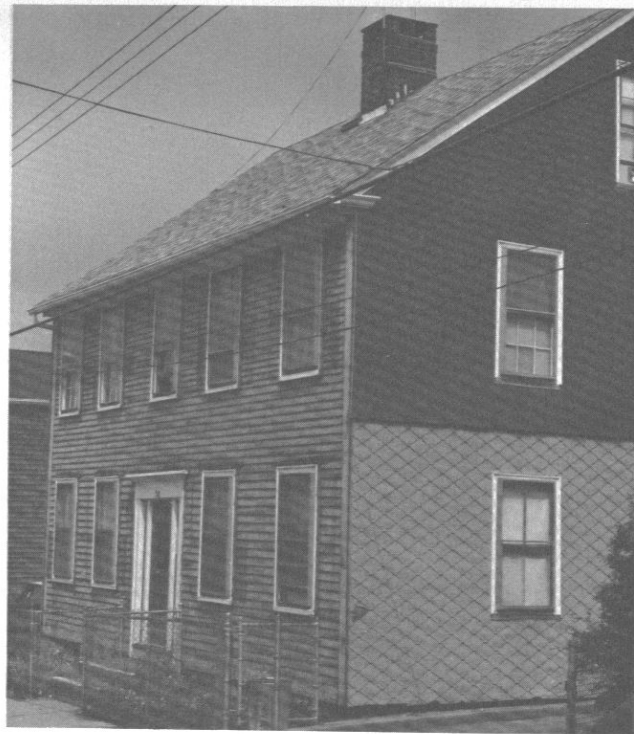
Fig. 49: 28 Pope Street (c. 1800), before restoration.
