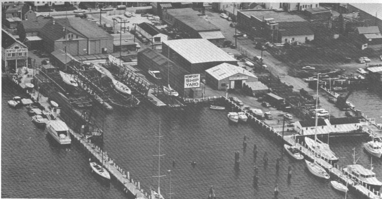
Fig. 25: Newport Shipyard, now Newport Offshore Ltd. This property has been a shipyard since 1834 when it was purchased by Silas Cottrell. In the mid-18th century merchant Josiah Brown's wharf was located here.
