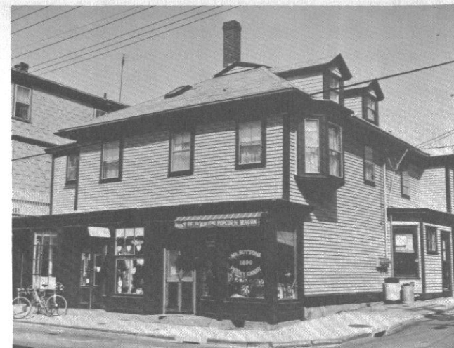
Fig. 29: James Carpenter House (c. 1765, with late 19th-century storefronts), 406-410 Thames Street.
