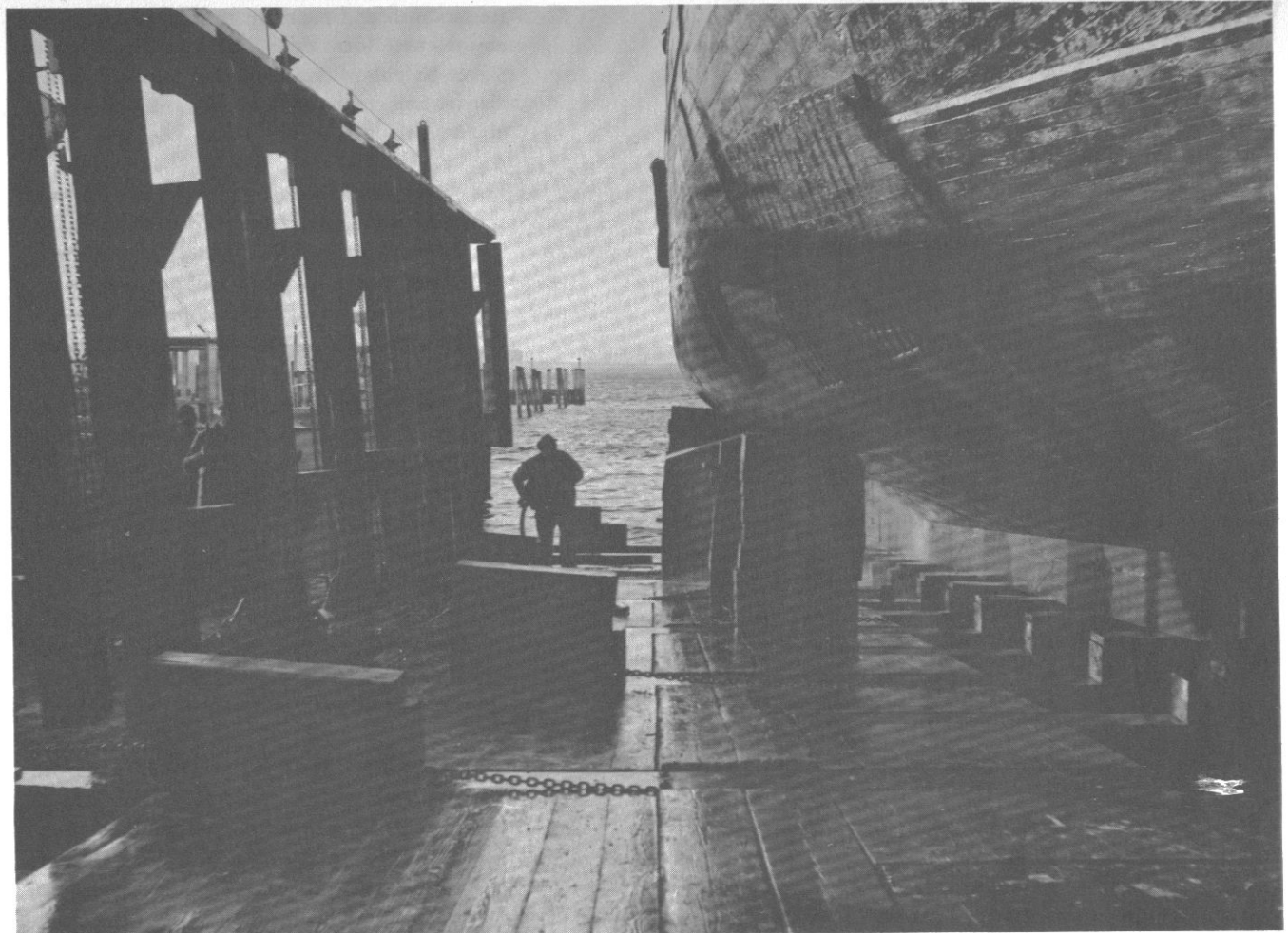
Fig. 60: West Howard Street Wharf; view west toward the harbor.
