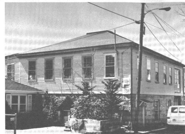
Fig. 58: 16 Coddington Wharf (the last surviving portion of the Coddington Mill complex) before renovation.
